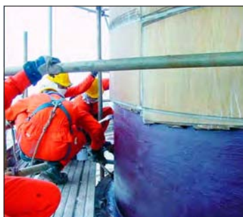
PROTECTION OF PROCESS VESSELS
