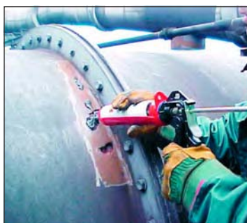
INFILL CORROSION PITS
