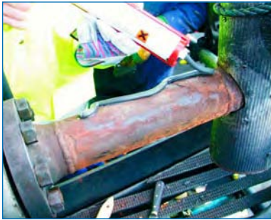
Belzona® 1251 - Rebuilding grade product designed to infill corrosion pitting and for bonding doubler plates over badly corroded areas.
